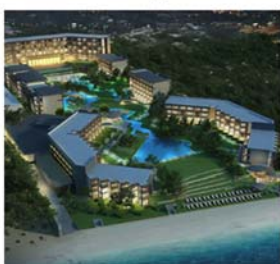
Marriott Hotel Renovation
