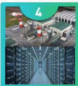
4 Power & Infrastructure Business
